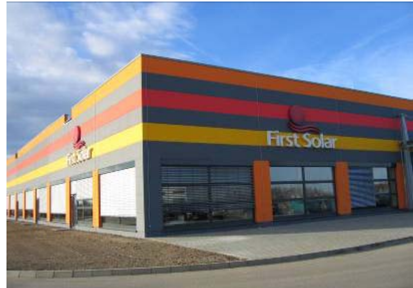
First Solar Manufacturing Plant, Frankfurt (Oder), Germany
