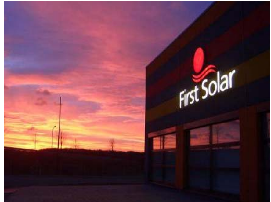
First Solar Manufacturing Plant, Frankfurt (Oder), Germany
